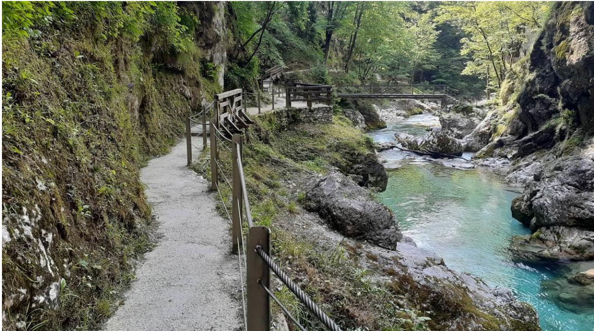
Photo 58. The iron handrail ensures the safety of walkers in dangerous areas in the Tolmin Gorges, Triglav National Park.
