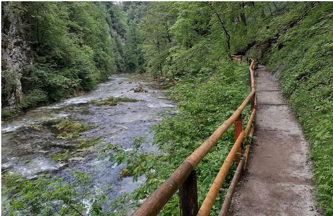
Photo 47. The wooden handrail ensures the safety of walkers and is in harmony with the environment in the Vintgar gorge, Triglav.
