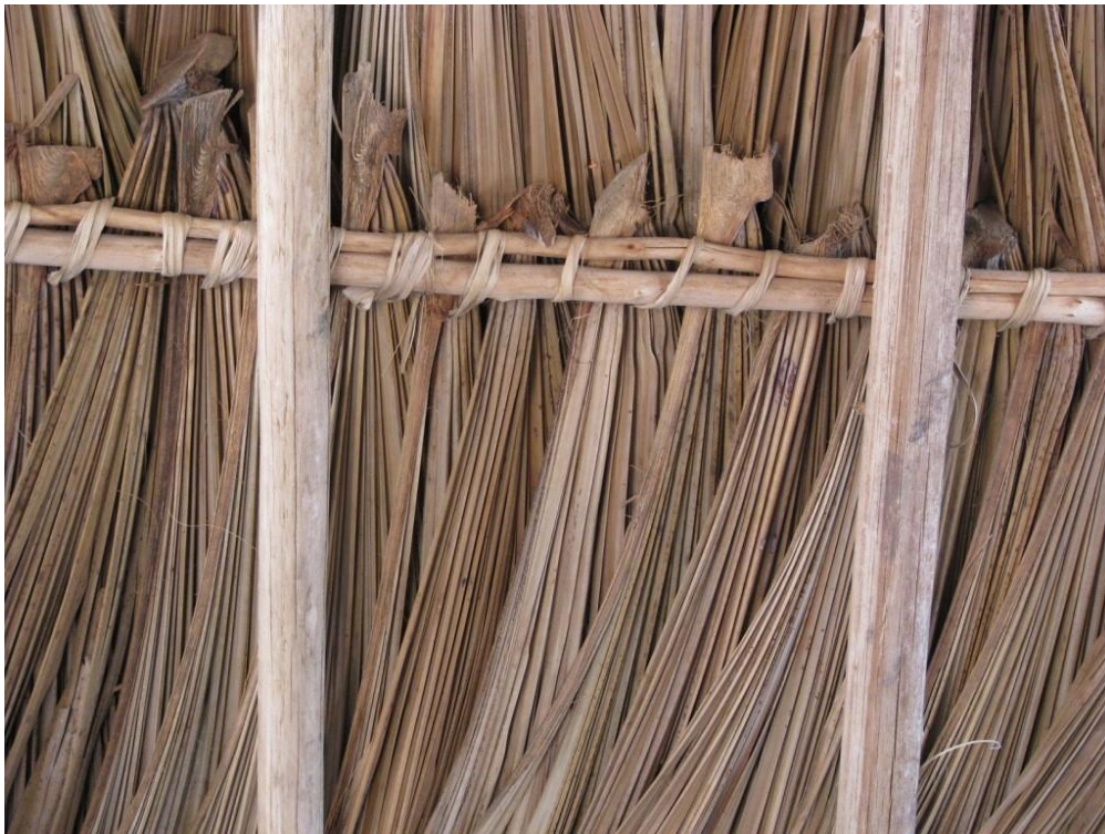
Photo 85. Detail of the Bororo house roof made of wood and buriti palm leaves ( Mauritia flexuosa ).
