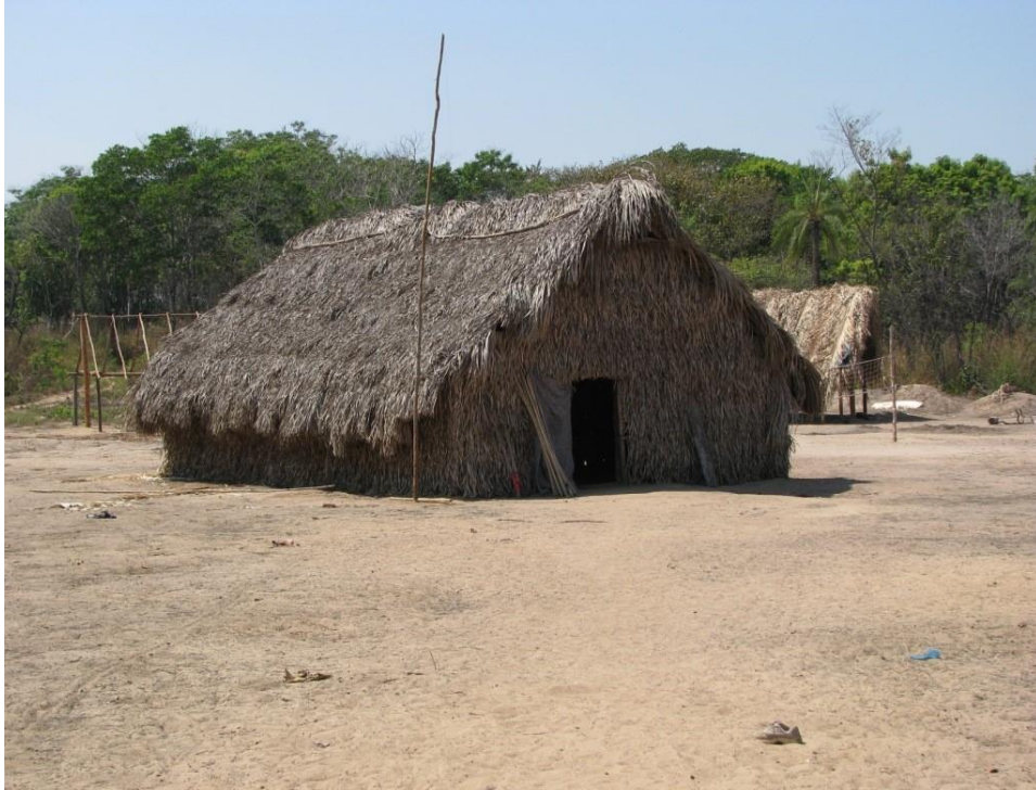
Photo 83. Bororo village house made of wood and covered with babassu palm leaves.
