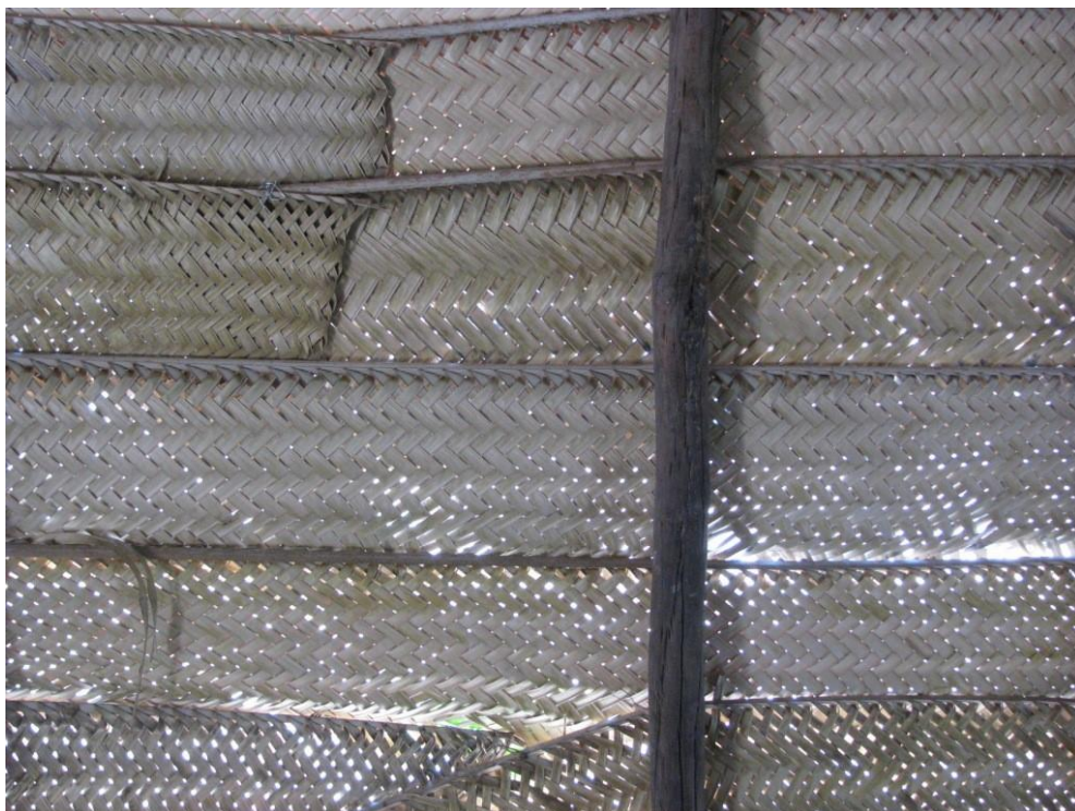
Photo 86. Detail of the Bororo house roof made of braided babassu palm leaves.
