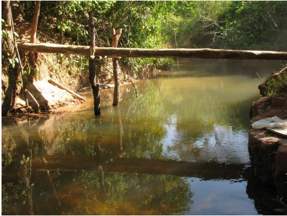
Photo 87. Bridge over a stream built from the trunks of a sturdy wooden wall tree, known by the Bororo by the name of ári ika ( Austroplenckia populnea ).
