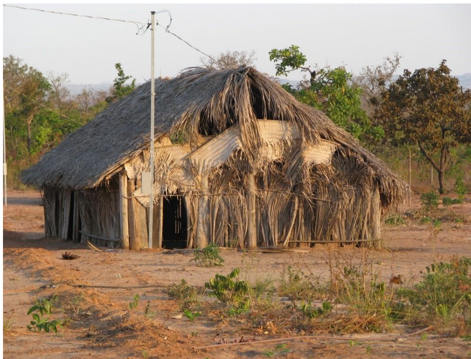
Photo 82. Bororo village house made of wood and covered with babassu palm leaves.
