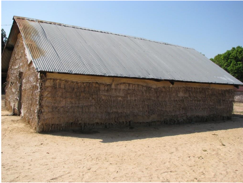
Photo 79. Bororo village house made of wood and babassu palm leaf ( Attalea speciosa ) and buriti palm leaf ( Mauritia flexuosa ). The roof is with metal tiles.
