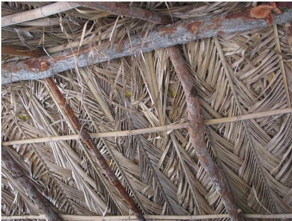
Photo 84. Detail of the Bororo house roof made of wood and babassu palm leaves.
