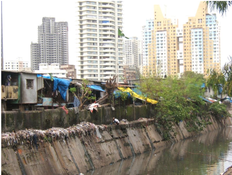
Figure 124. Cluttered Bombay/Mumbai City
