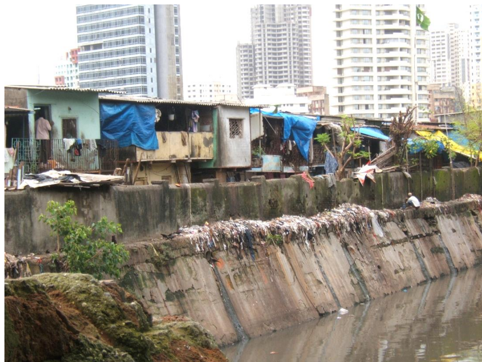
Figure 125. Cluttered Bombay/Mumbai City
